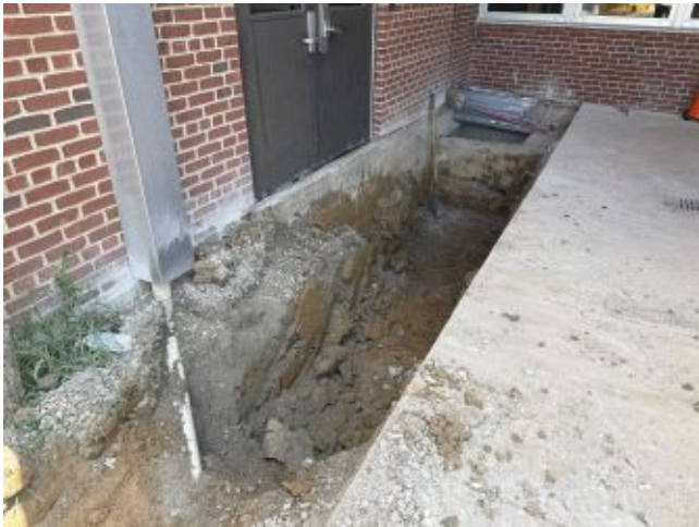
2026.07.30 – Trench for geothermal entry into building
