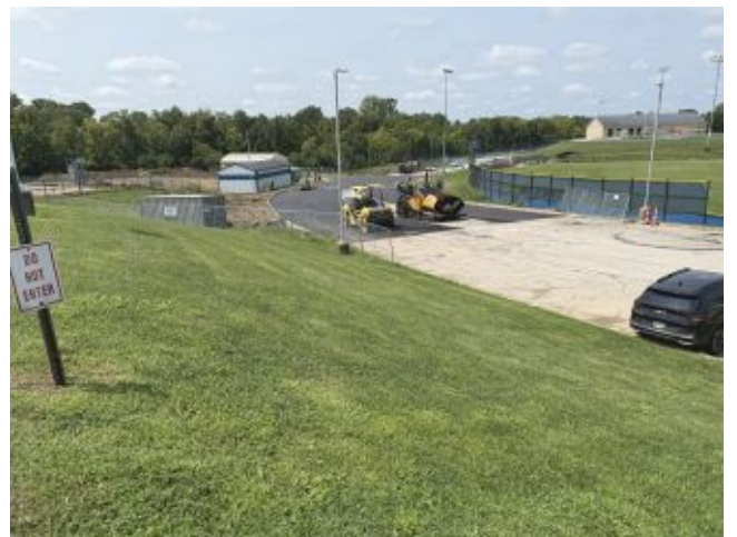
2026.08.13 – Paving SK parking lot
