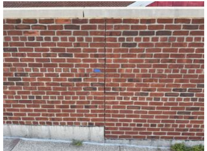
2026.07.30 – Cut out CJ ready for caulking
