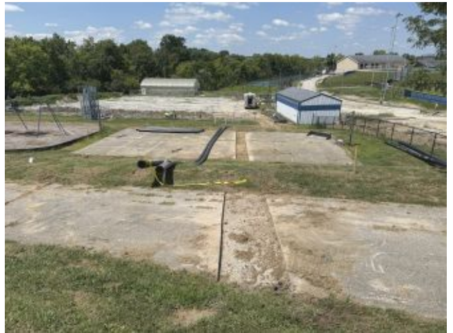
2026.07.30 – Pathway for geothermal to the building
