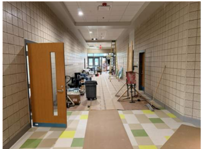
2026.08.11 – New addition main entry corridor
