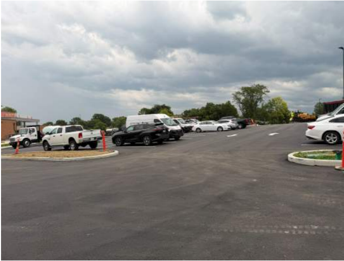
2026.08.11 – West parking lot new paving
