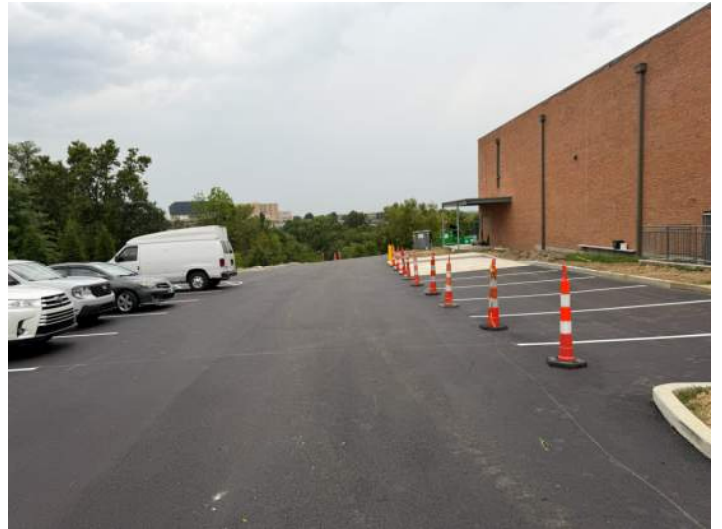
2026.08.11 – West parking lot new paving
