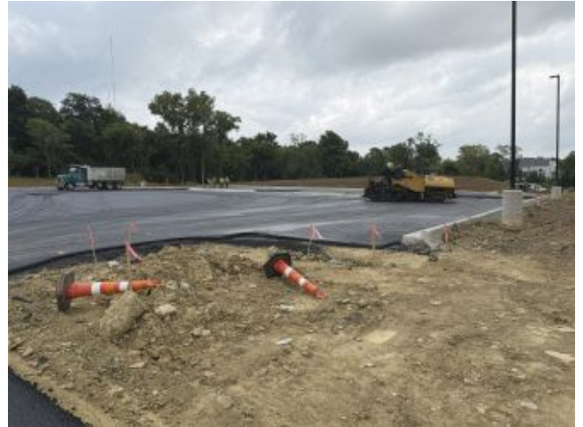
2026.07.28 – New parking lot
