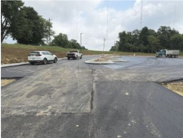
2026.07.28 – New parking lot
