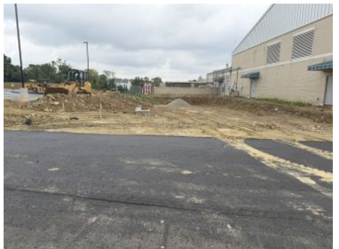
2026.07.28 – Looking towards loading dock
