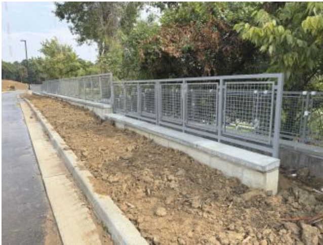
2026.08.11 – Guardrail at new retaining wall
