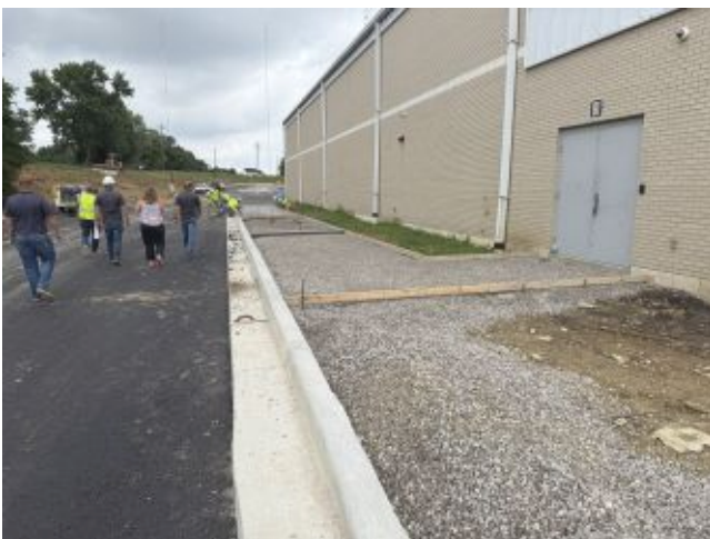
2026.07.28 – West side of gymnasium
