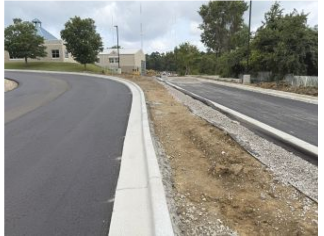
2026.07.28 – Drive along east side of building
