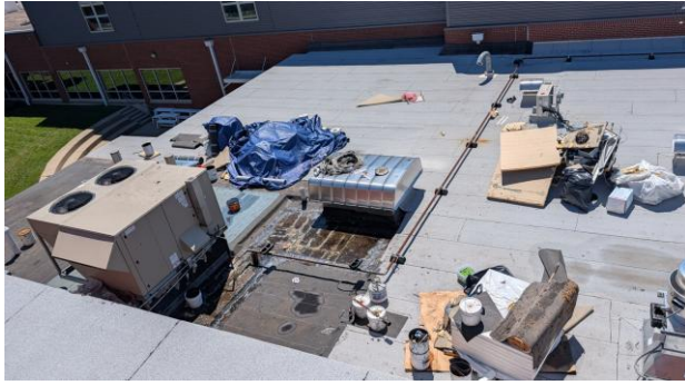
2026.08.18 – New modified bit roofing system and insulation installation above Boiler Room and Kitchen
