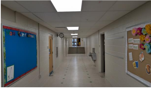
2026.08.18– Corridor #104 looking north
