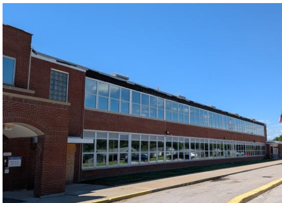
2026.08.18 – Exterior work on North Elevation
