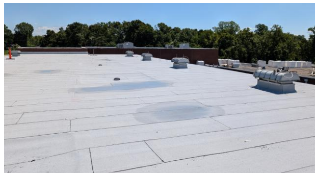
2026.08.18 – New modified bit roofing system and insulation installed above Classrooms
