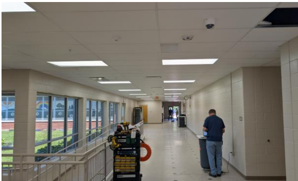
2026.08.18– Corridor #132 looking north
