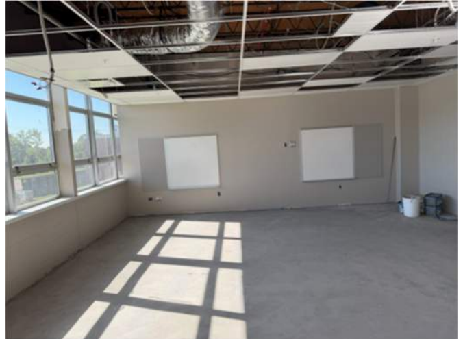
2026.08.18 – Typical Phase 1B classroom
