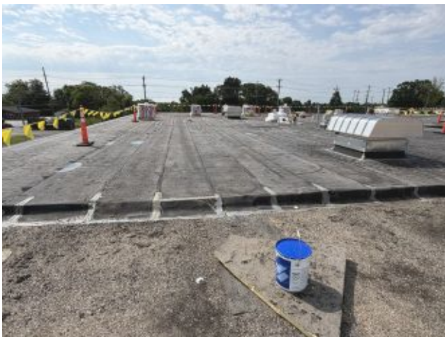
2026.08.06 – Roof over Phase 1A
