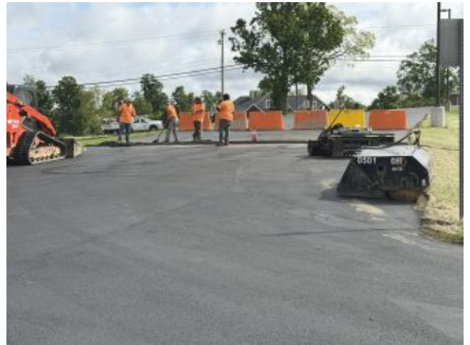
2026.08.20 – Installing speed bump on queue drive
