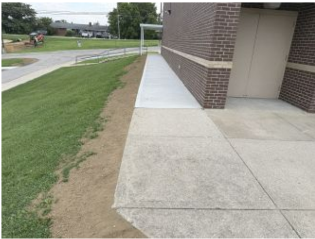
2026.08.06 – New gym sidewalk with topsoil
