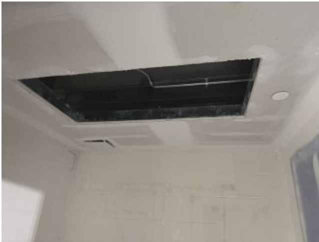
2026.08.06 – Blue Room ceiling
